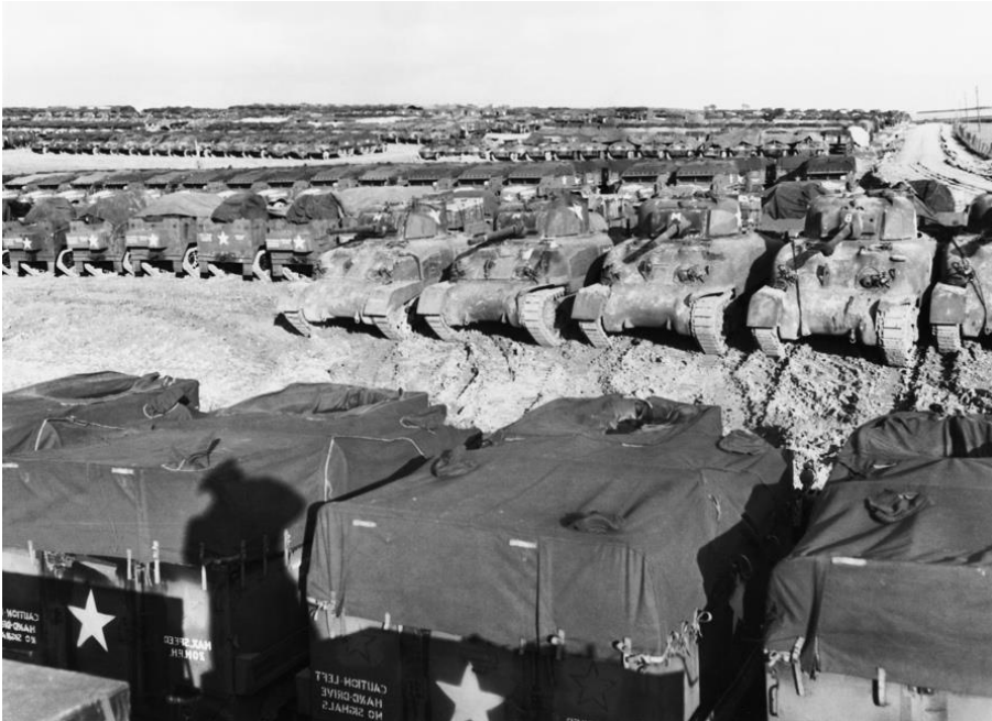
Vehicles being stored © SC 187235
